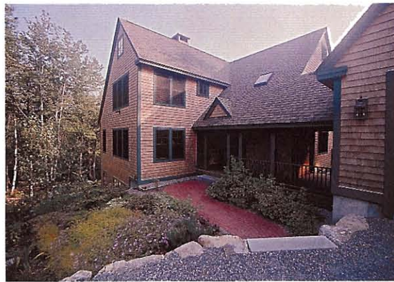
This brick pathway with native plantings, makes this entry a pleasure to come home to.
